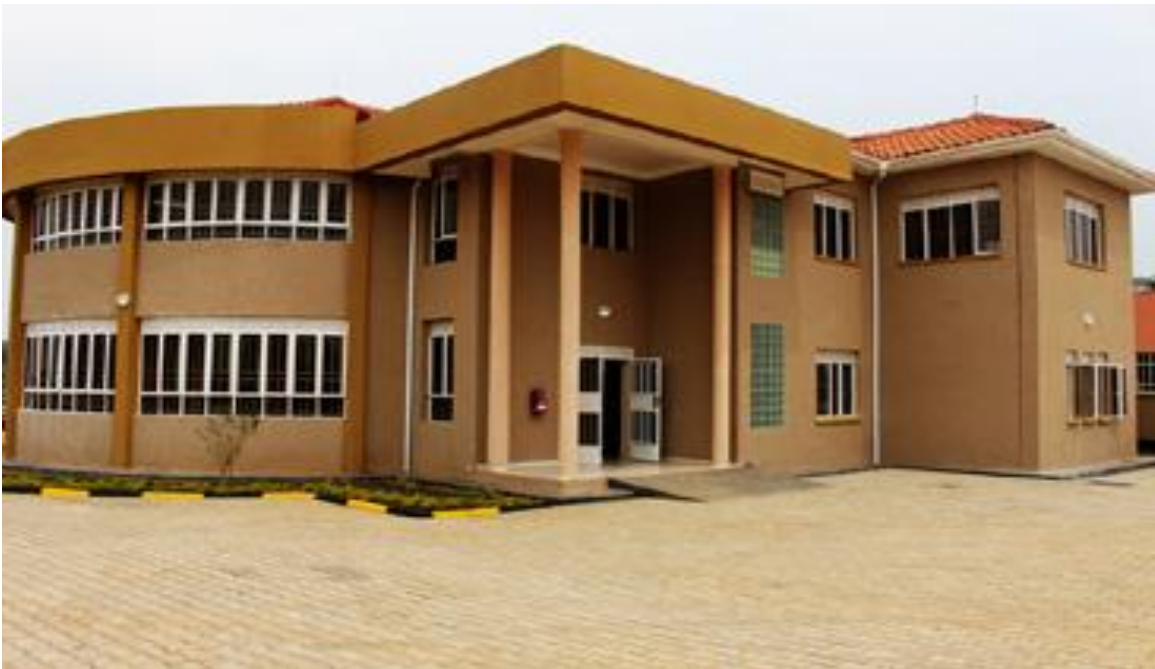
The newly commissioned Mbarara Branch Office
