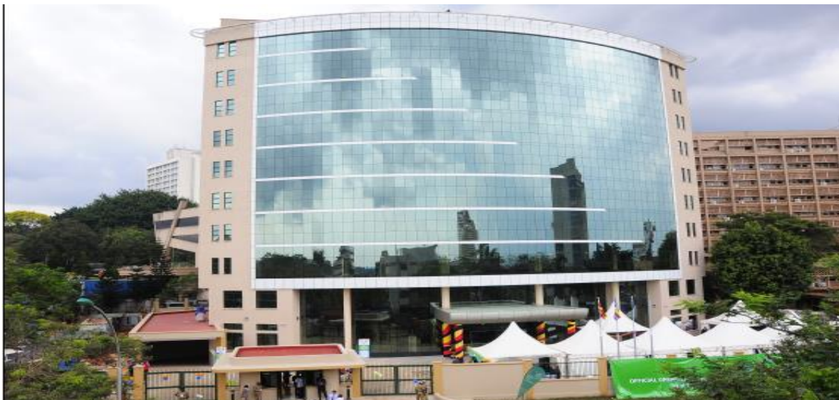
The newly commissioned Audit House. Headquarters for Office of the Auditor General in Kampala
