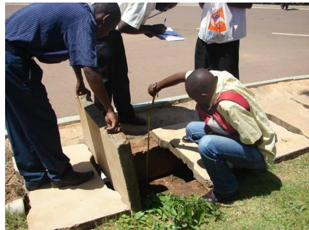
Picture 20: Munyonyo CWR driveway and parking. Measurement of lined drains and covers 620×970×75mm. (Dott Services/ MoWT)
