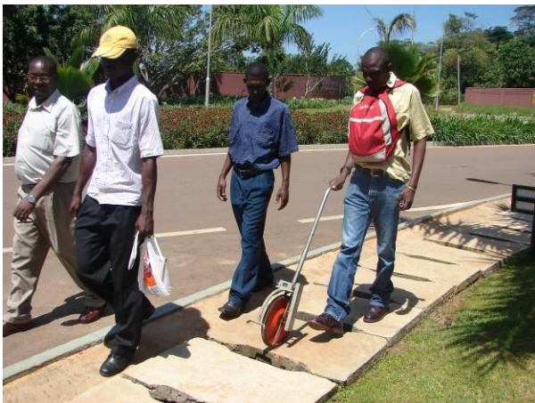
Picture 19: Munyonyo CWR driveway and parking. Note lined drains and covers 620×970×75mm. (Dott Services/ MoWT)
