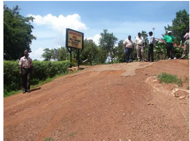
Picture 27: 2 nd sealing at road junctions. Salaama Rd.. (Dott Services/ MBW)
