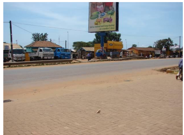
Picture 4: Guardrails damaged by accidents at Abaita Ababili market on Zana - Entebbe Rd. Regular maintenance needed. (EnergO Ltd/ MBW)
