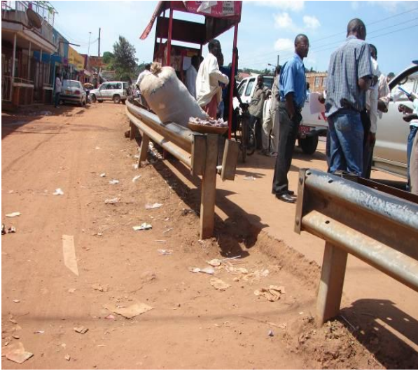
Picture 28: Counting of guardrails at Kajjansi on Zana - Entebbe Rd. (Energo Ltd/ MBW)
