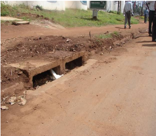
Picture 16: Poor drainage maintenance. Jinja Rd near Lugogo Indoor Stadium (Cementers/ PROME)
