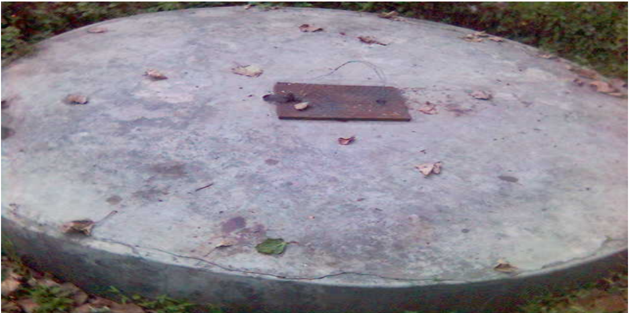
The placenta pit was built at a site with a low water table causing it to be water logged
