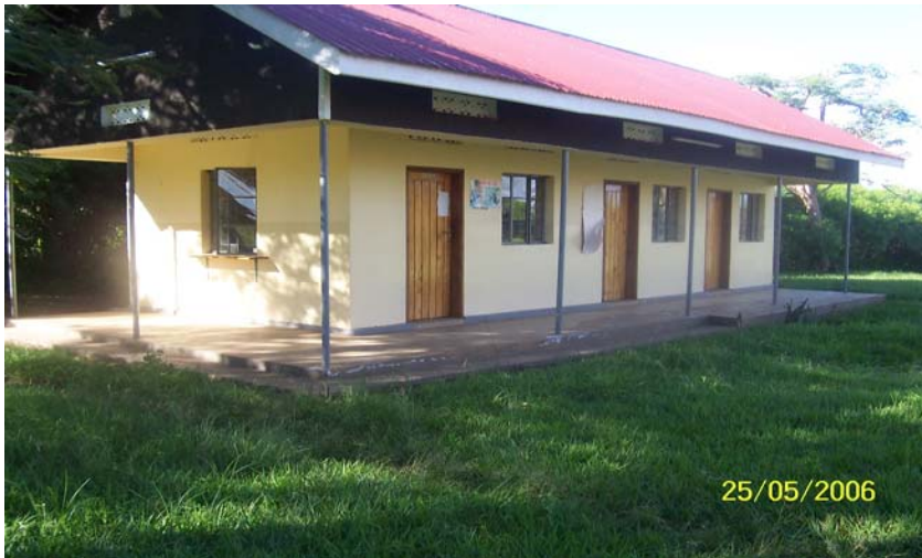
A building for HCT that was constructed through funding by UACP in Mukono District
